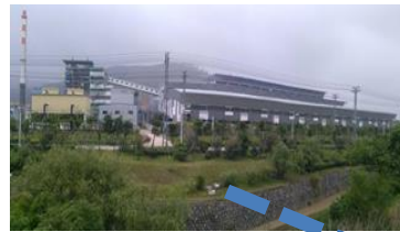
Food waste recycling plant
